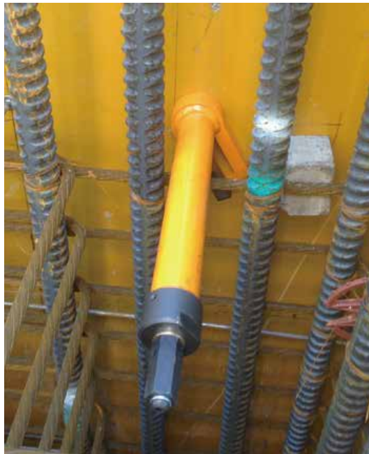
※ Replacing the spacer.
