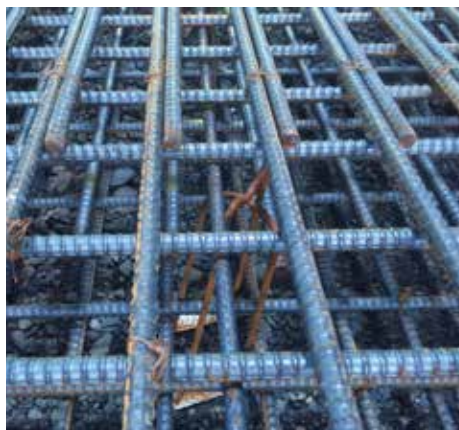
※ Replacing the spacer.
