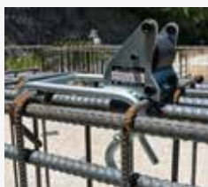
Put on to the rebar
